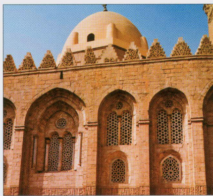
Above The Mamluk Sultan Qalawun built this mausoleum in 1285 as part of his much larger complex in Cairo, Egypt.
