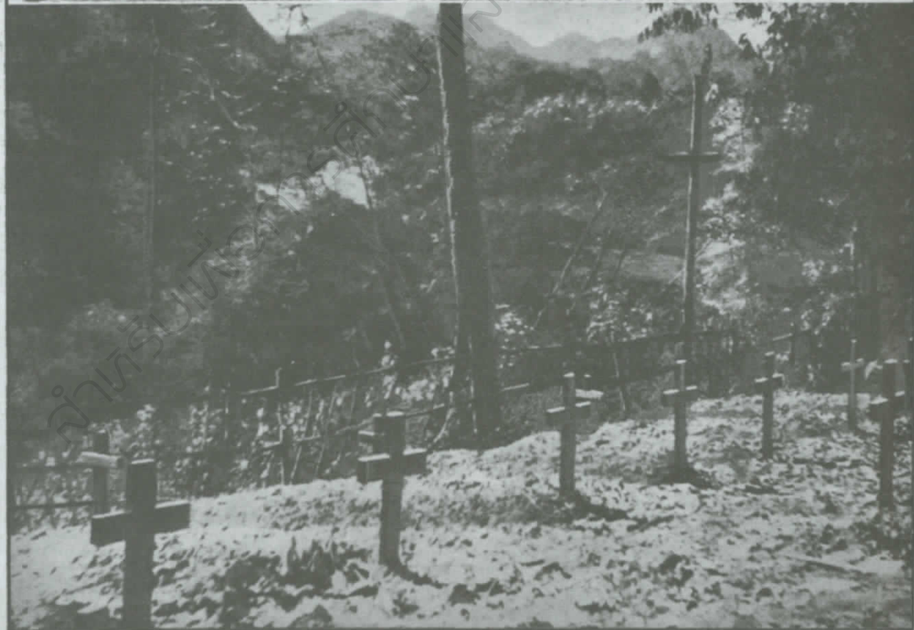
A SINGLE TRACK FROM SIAM TO BURMA, the notorious Bangkok-Moulmein railway (top) was constructed under compulsion of the Japanese by British and Allied prisoners of war and 100,000 native labourers, in 1942-43. Toiling for 17 hours a day in appalling conditions, in disease-ridden and pest-infested jungle, men died like flies: their last resting-place line-side cemeteries such as this (bottom) recently cleared by Jap gangs under Allied supervision. See also story in page 409.
