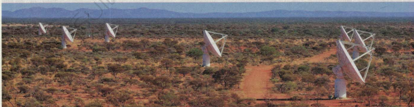
The Australian Square Kilometer Array Pathfinder consists of 36 separate dish antennas spread across a wide area, working together as one. It can detect millions of other radio signals in a matter of days, and found 20 FRBs in 2018, almost doubling the current total.
